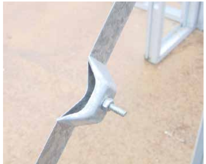
Figure 7.23 use tensioner on strap bracing to bring the wall into square.
