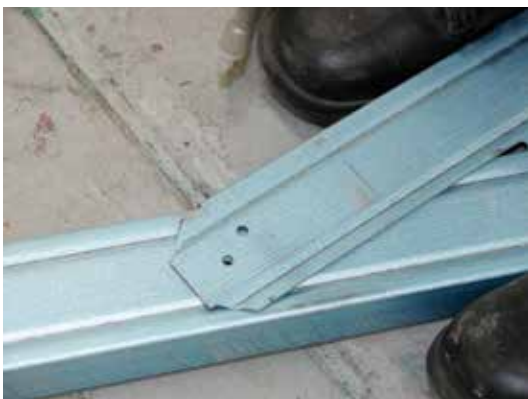
Step 3 - Align holes, fix at heels and install a locating truss screw
