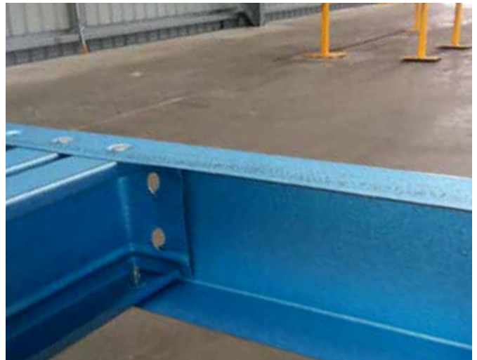
Figure 6.22 Twist stud into position & align fixing holes – repeat for all studs along bottom plate.
