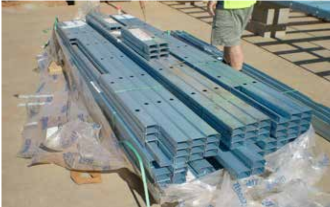
Figure 6.8 Wall frames are individually strapped & stacked in “stud” bundles, labelled with bundle numbers
