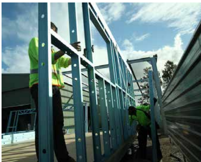
Figure 7.4 Place first wall on marked line and hold in position.
