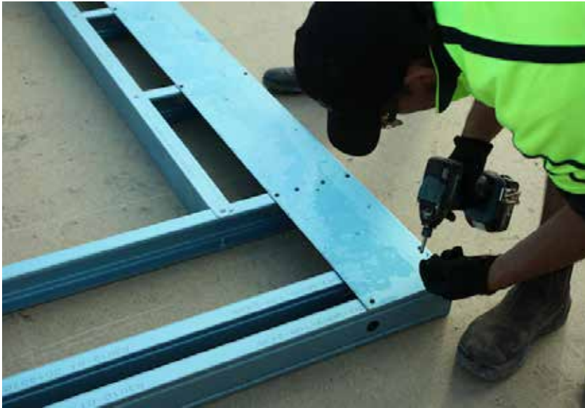
Figure 6.36 Overlay & screw fix lintel flashing to top of frame as per assembly sheet & fixing details given in the Design Manual. (Refer below)
