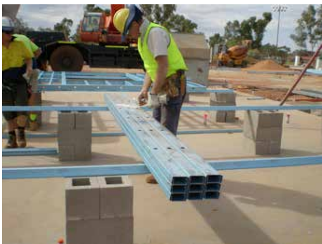
Figure 6.14 Lift & separate stud pack onto assembly table (this example has utilised TOPSPAN® 40 sections on concrete block stacks as an assembly table).
