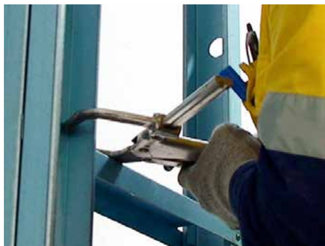
Figure 7.12 Use clamp to hold temporarily in position.
