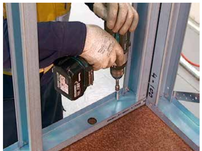
Figure 7.20 Screw bottom plate into final position on floor.
