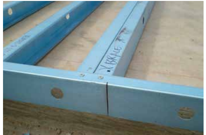
Figure 6.33 Marking frames
