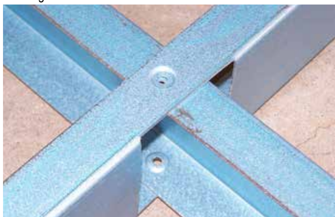
Figure 6.28 Nogging Installation
