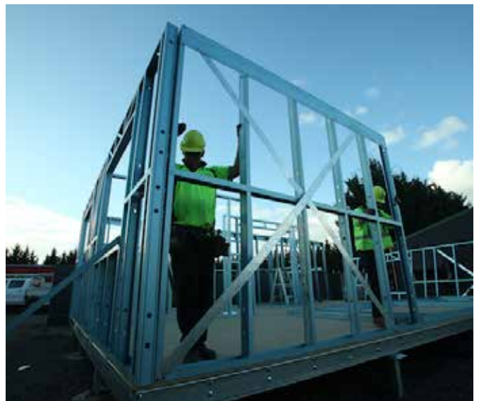
Figure 7.9 Structure with temporary bracing.
