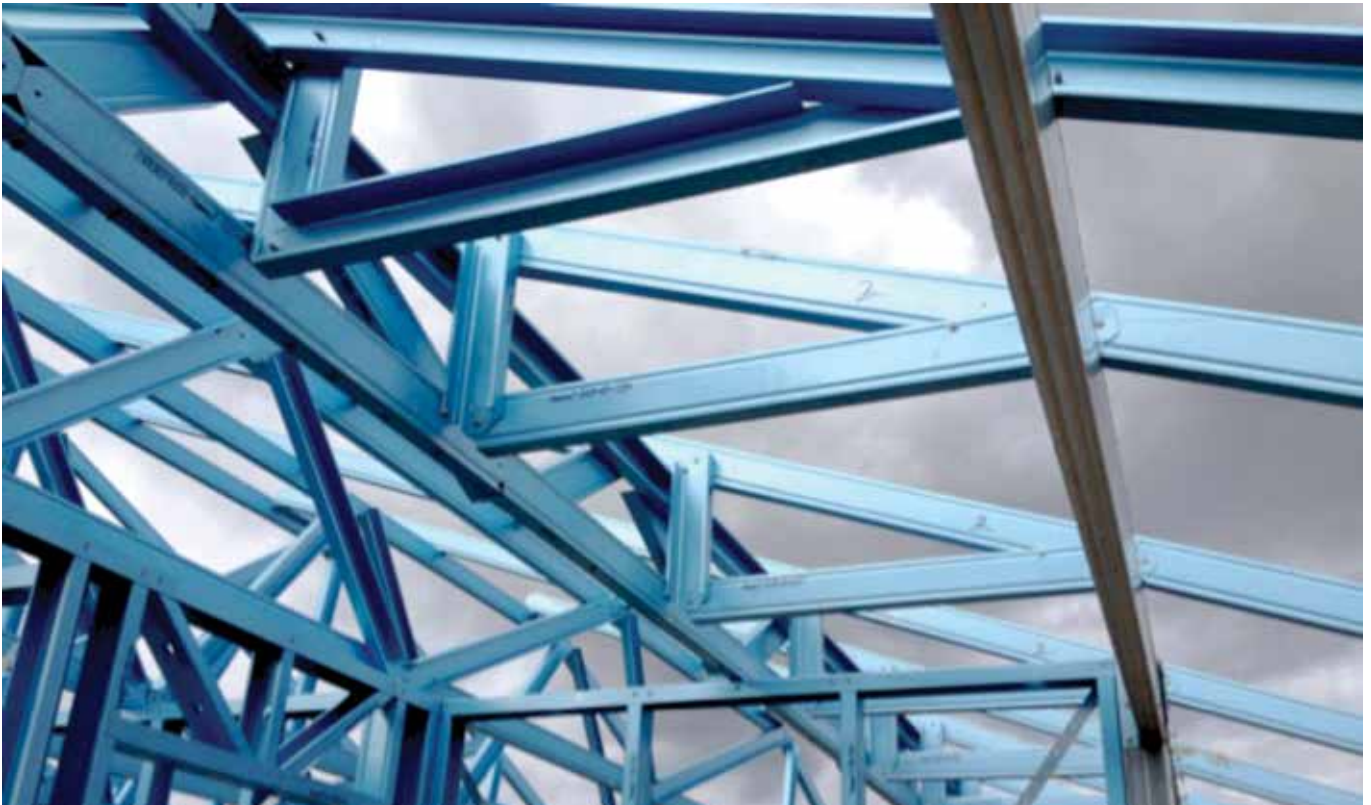
Figure 11.8 Installation of a Type 1A hip truss
