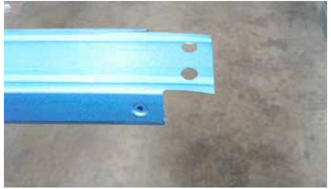
Figure 6.20 Prepare tabs and align with top of studs & screw fix top plate at both ends. (Where utilised, ensure Endurotie™ bent tab studs are placed in the correct location and orientation.)
