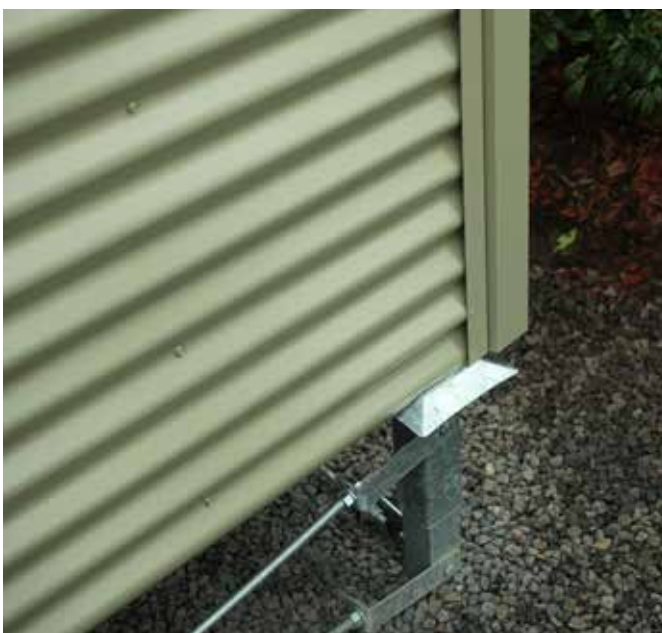
Figure 7.44 Sheet trim flashing at corner locations
