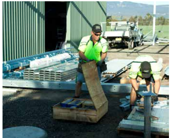
Figure 6.11 Sort & stack all accessories, cross check packing list. (helps to mark on box's, where accessories are to be used)
