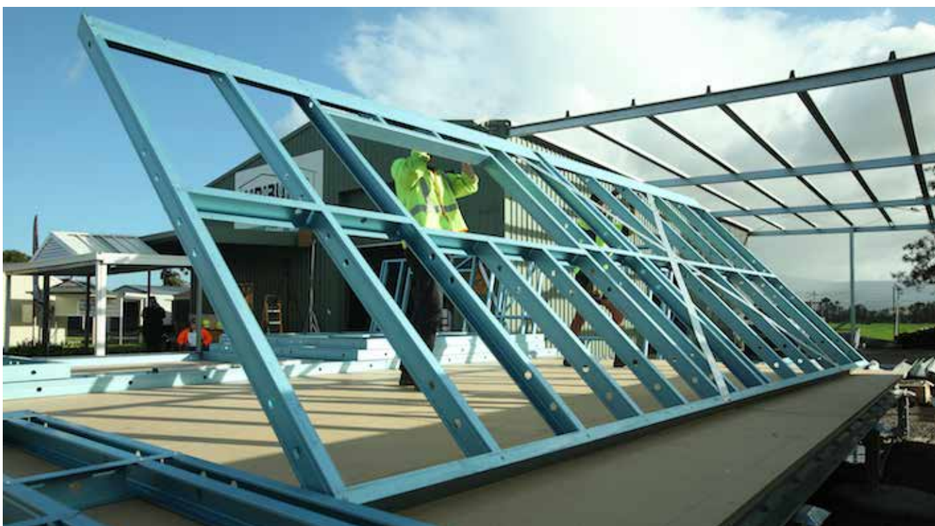
Figure 7.4 Place first wall on marked line and hold in position.
