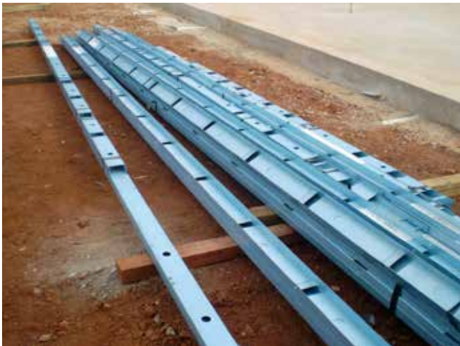
Figure 6.9 Matching frames in “hogging, top & bottom plate” bundles, labelled with bundle numbers
