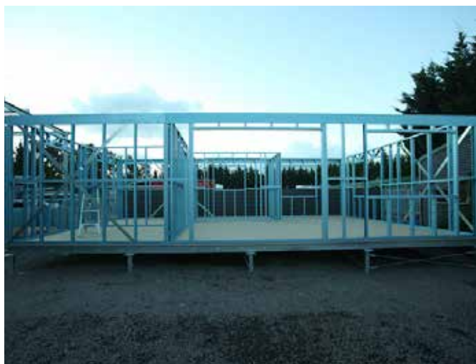
Figure 7.11 Interior walls are fixed into position.
