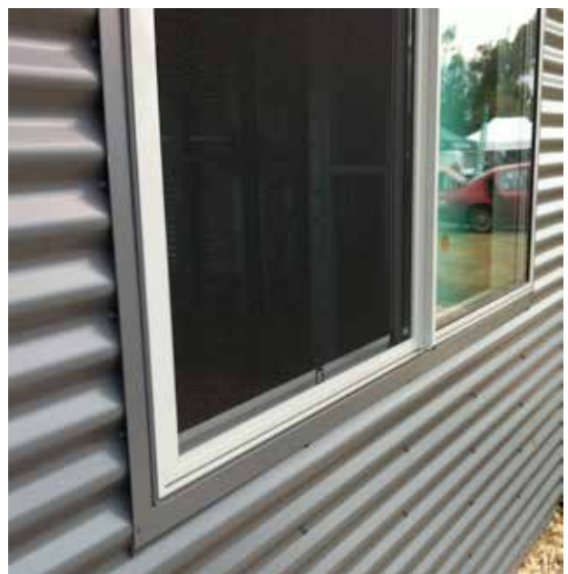
Figure 7.45 Sheet trim flashing around window and doors
