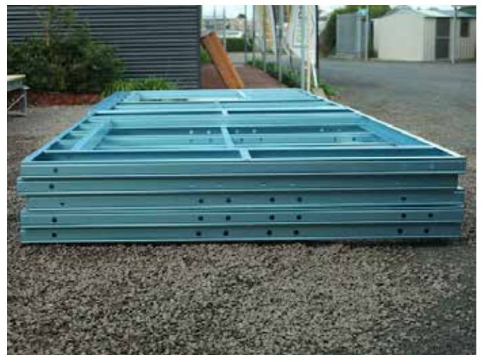
Figure 6.41 Stack wall frames in bundles close to the final installation position.
