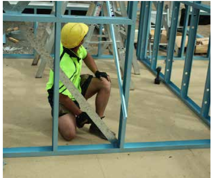
Figure 7.8 Affix temporary bracing as required.
