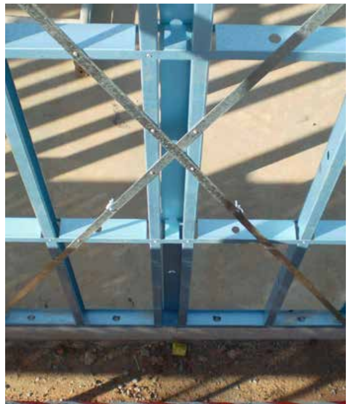
Figure 7.24 Check plumb and square and adjust as required.
