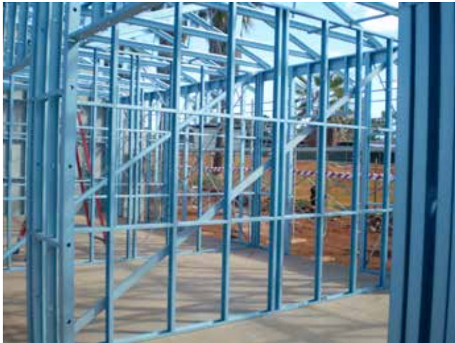
Figure 7.15 Position final wall.
