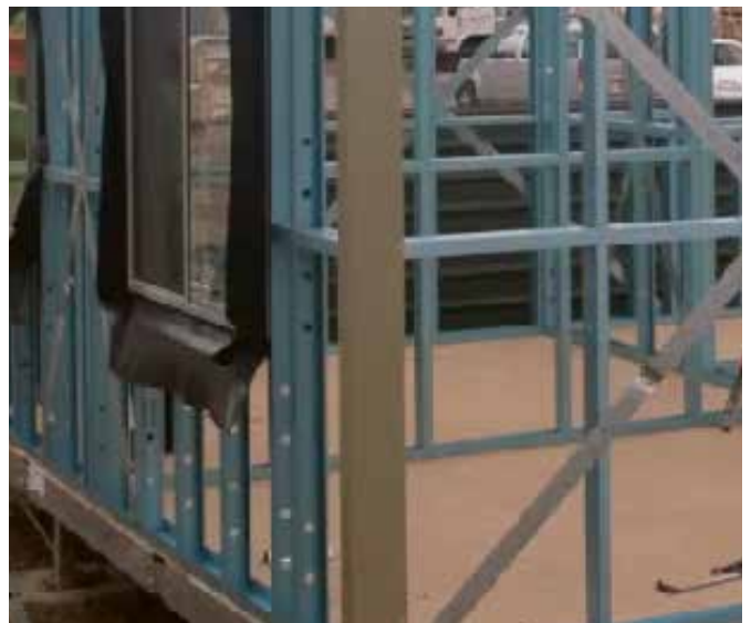
Figure 7.43 Preliminary flashing for the corners of the building
