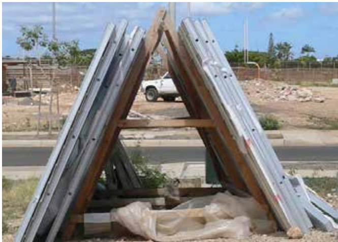
Figure 2.1 Frames stacked vertically
