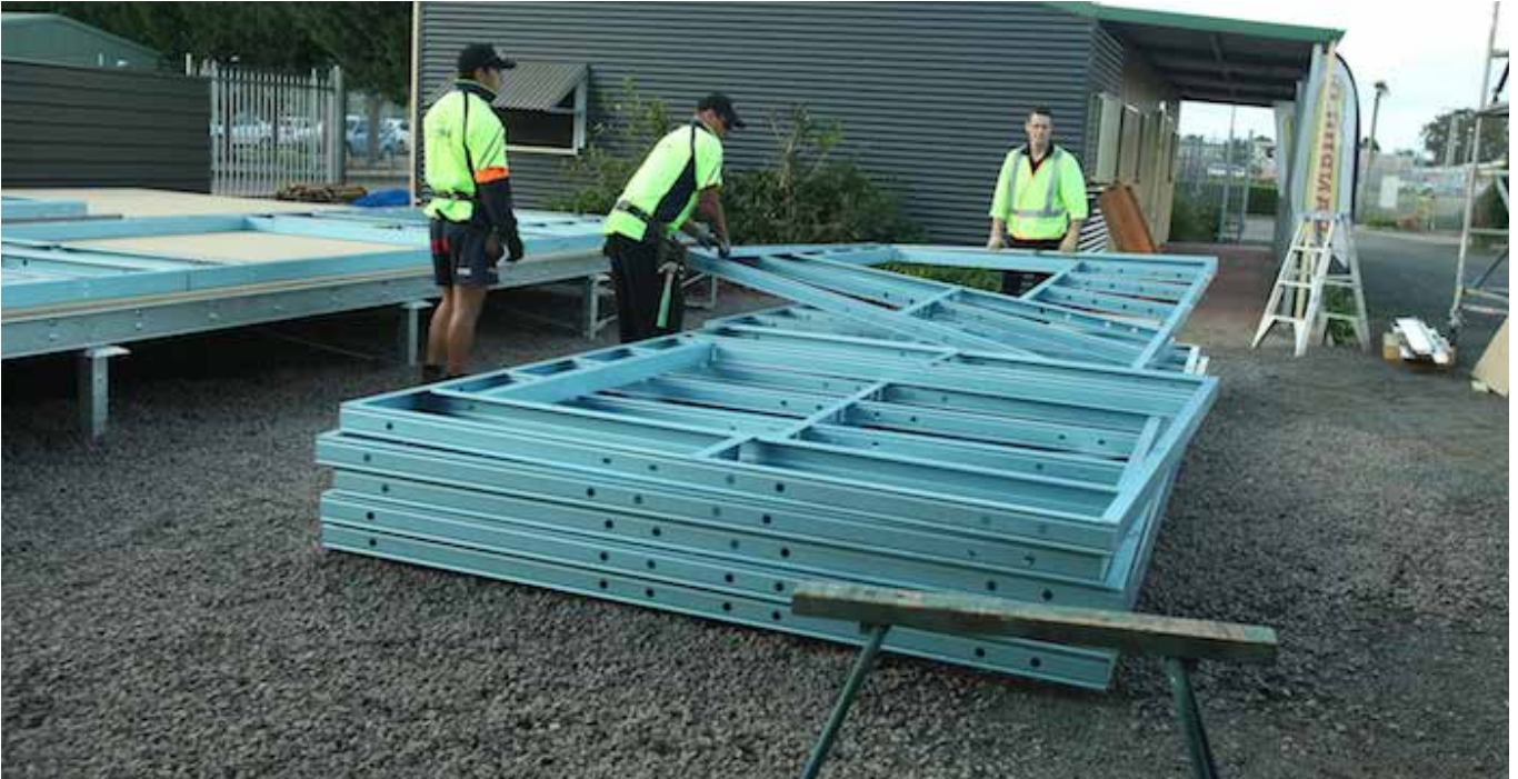
Figure 6.39 Relocate completed frames to a designated stacking area.
