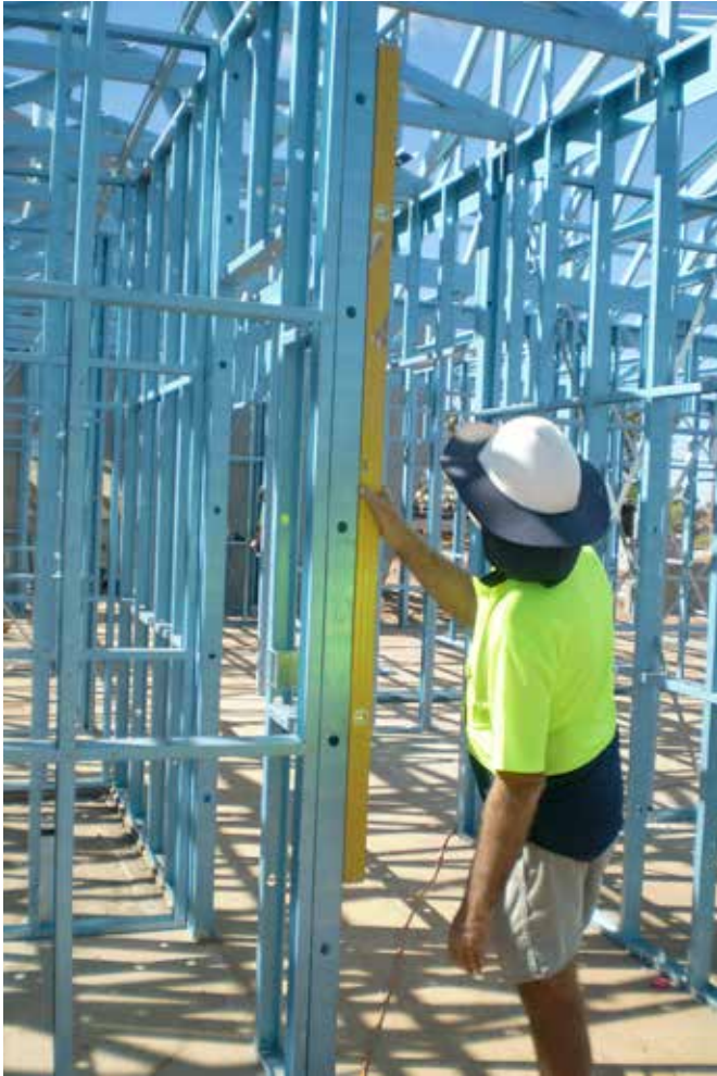
Figure 7.21 Check walls for plumb.
