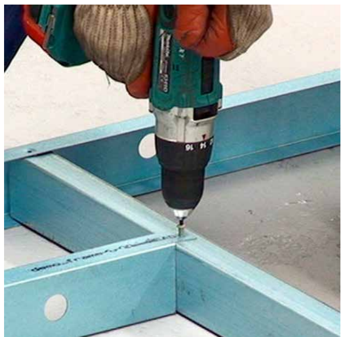
Figure 6.24 Align notch holes as shown and install M6x1Px15mm smooth top fastener in holes.
