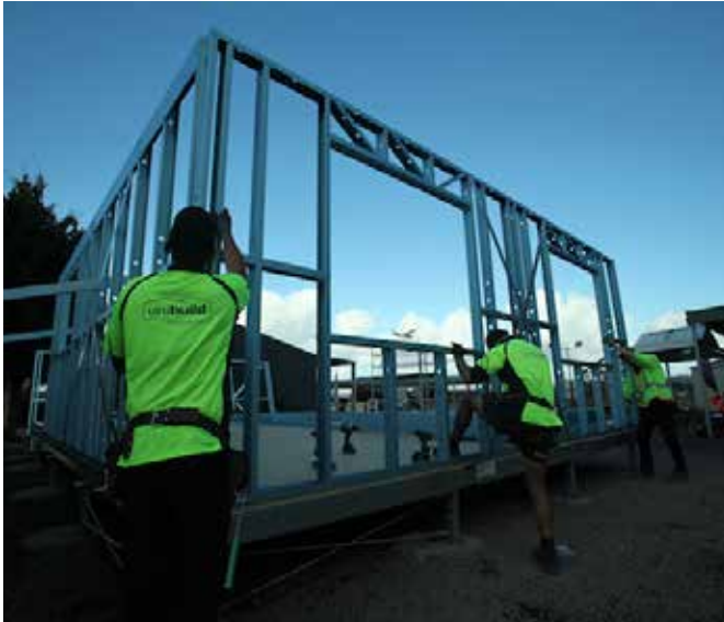
Figure 7.5 Place second wall in position using chalk line as a manual and flush against first wall.
