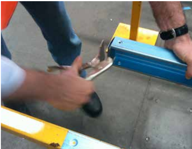
Figure 6.21 Bend tab over and fix all studs by inserting into bottom plate on approx. 45° (degree) angle.
