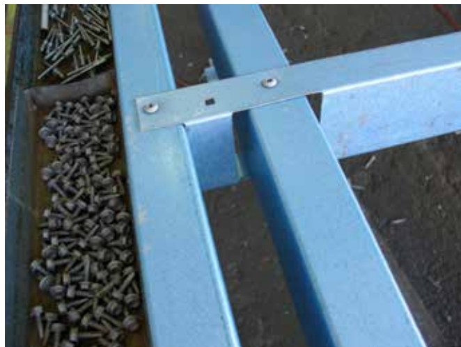
Figure 6.26 Nogging installation.
