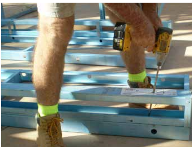
Figure 7.17 Join walls at corner using extension bit.
