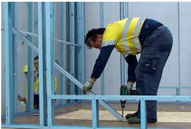
Figure 7.16 Remove last of the temporary bracing.
