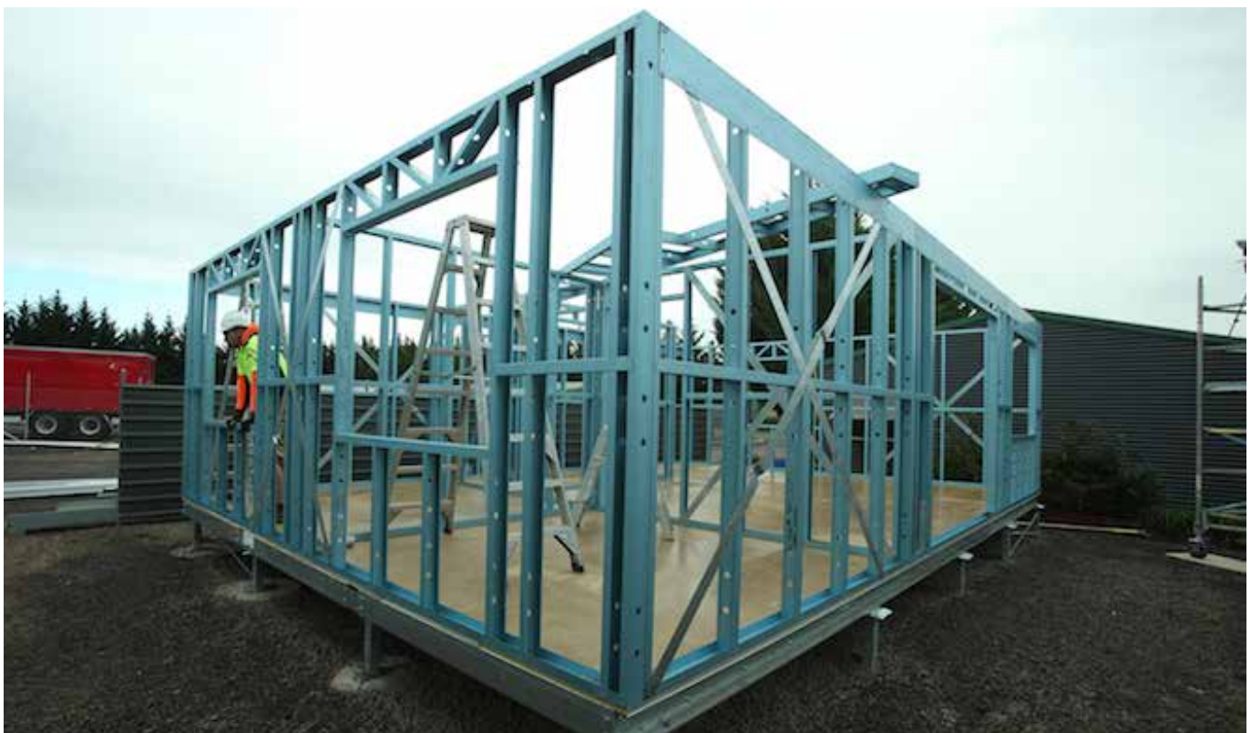
Figure 7.28 Wall up, plumbed, squared and fixed - ready to fit roof trusses
