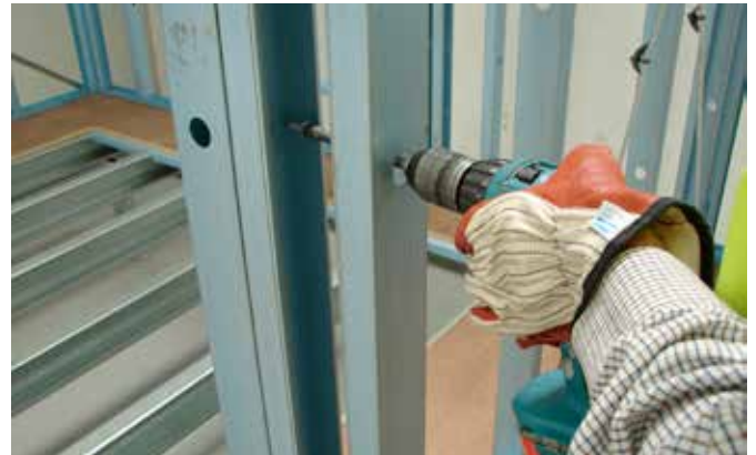
Figure 7.18 Position and fix final wall using extension bit.
