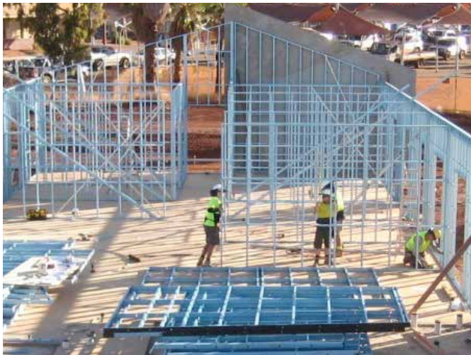
Figure 7.10 Place interior walls using chalk lines as manual.
