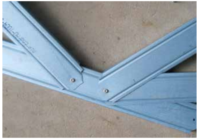
Finished knee web connection (unreinforced)
